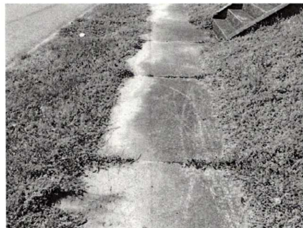
US 31W South Towards SR 76-Typical Pathway
