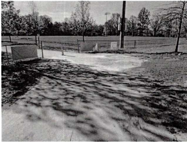
W.L. Anderson Sports Complex-Sidewalk Maintenance
