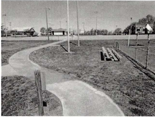
WH Mun. Park-Field 1-4 Sidwalk, No Access to Bleachers
