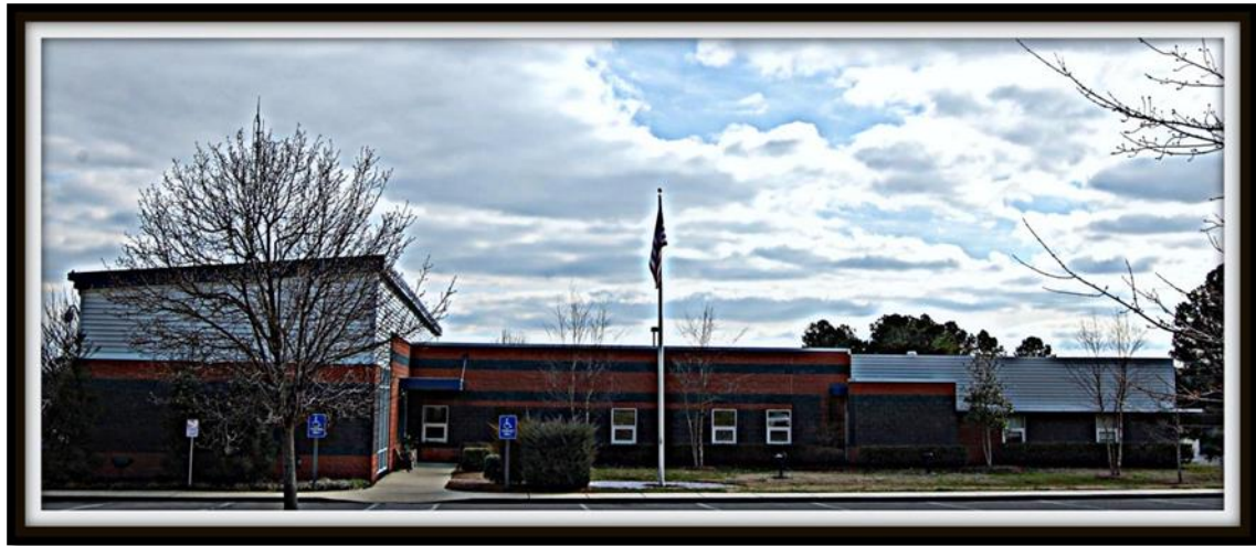
John W. Decker Police Facility
