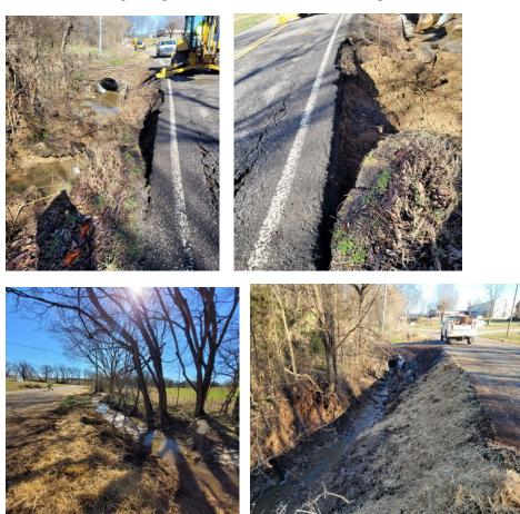
$\frac{2/15/2024}{1}$  Morgan trace – Drainage mitigation. Remove valley gutter causing traffic complaints and installed smaller gutter with drain.
