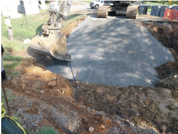
WO062323002 Capital improvement project at Village Court
