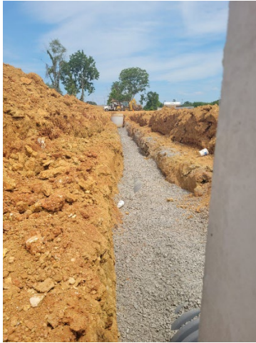
WO061323004 Inspection at the Mill's
