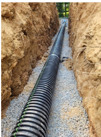
WO060823007 The Mill's inspection
