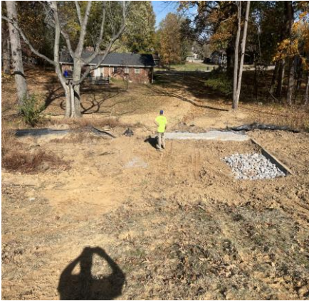
11/14/2023 – The Mills outfall modifications.
