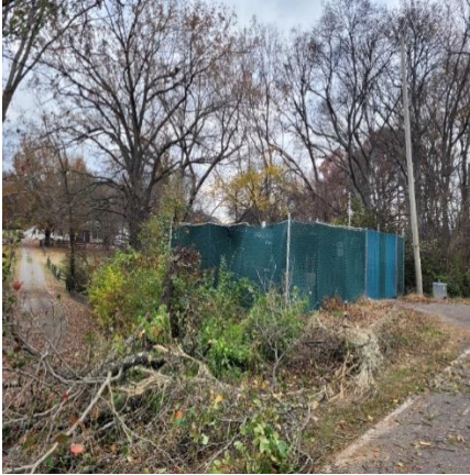
11/20/2023 - Storm cleanup at pump station
