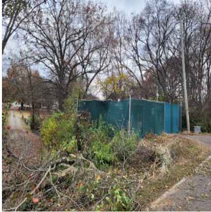
11/20/2023 - Storm cleanup at pump station
