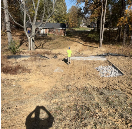
11/14/2023 – The Mills outfall modifications.
