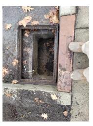
11/16/2022 WO111422004 412 Artesia Dr Drainage system was built up with debris and system made its own path and needed to be reshaped and hole filled in.
