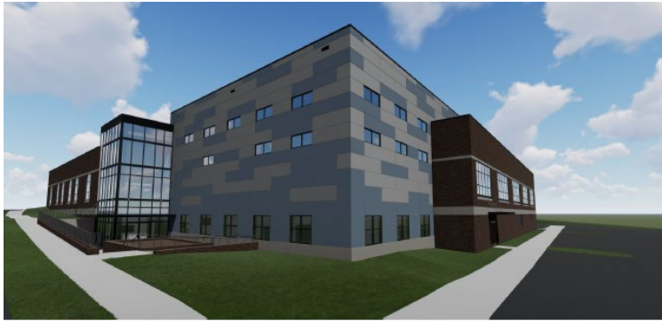
EXTERIOR - SOUTH WEST CORNER
