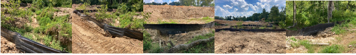
081722010 – Construction Site EPSC inspection: Summerlin: Reviewing twice weekly inspection for repairs.
