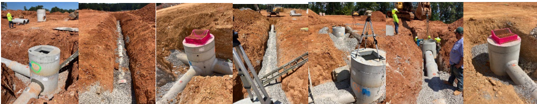
081722005 – Proof Roll: Copes Crossing Sub-grade: Inspection of compaction with a scaled load.
