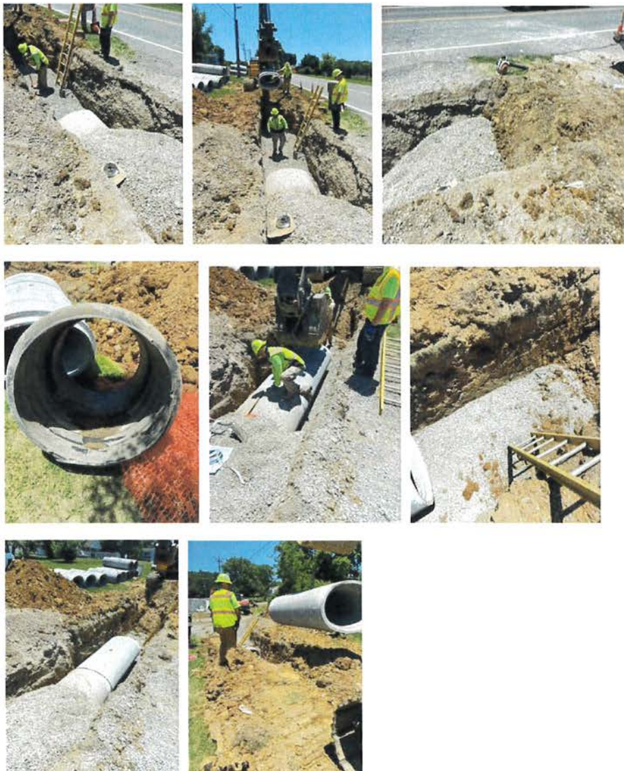
June 20 – Wilkinson Drainage Project
