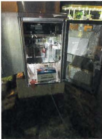
June 16 – Battery Back-up installation. SR-76 and Hwy 31W
