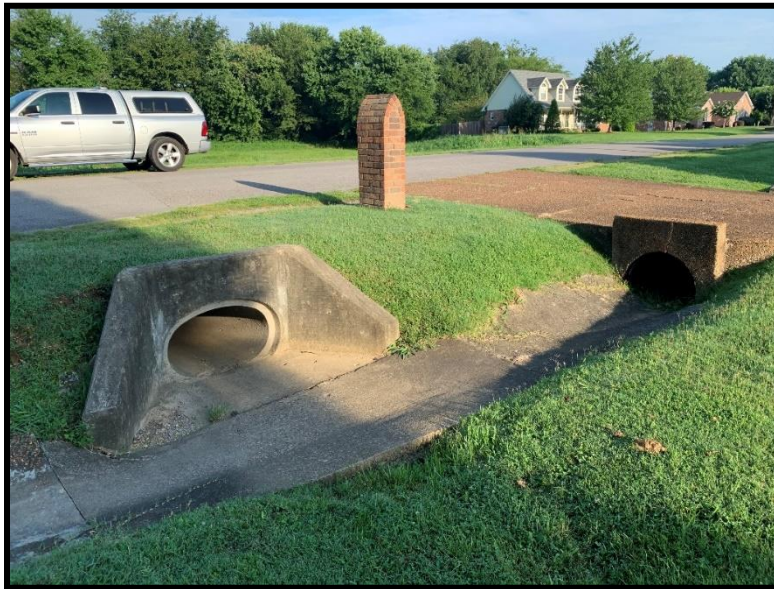
Figure 5: Existing 38"x24" Elliptical RCP Culvert Crossing Shady
