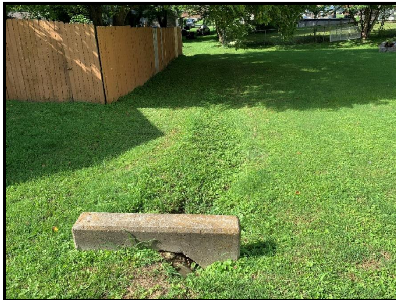
Figure 4: Existing 24" CMP and Ditch near Meadow
