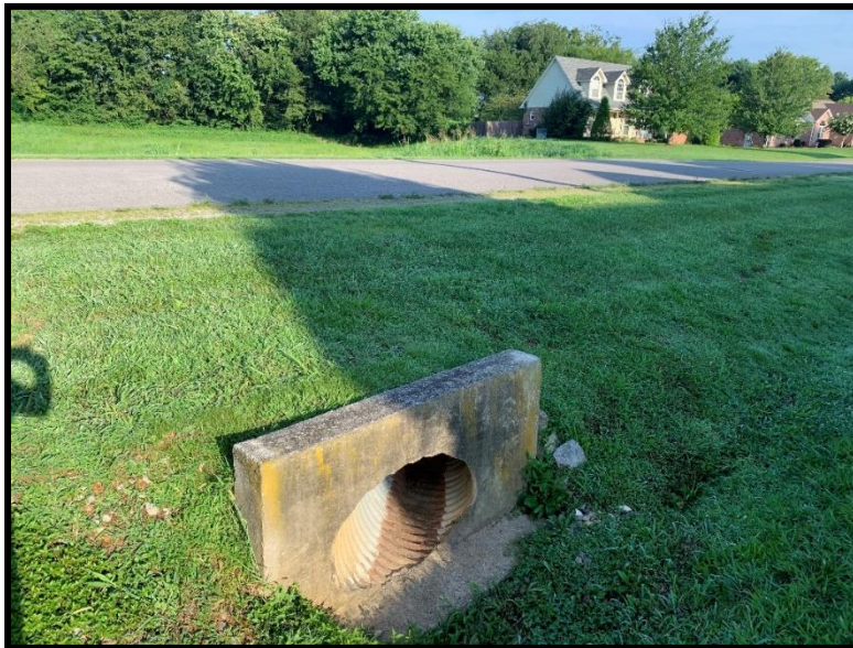
Figure 6: Existing 24" CMP Crossing Shady
