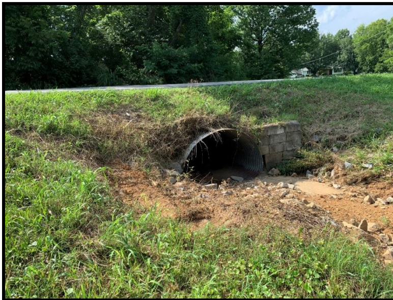
Figure 2: Existing 64"x43" CMP Arch Culvert Crossing Wilkinson
