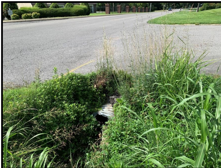
Figure 2: Existing 64"x43" CMP Arch Culvert Crossing Wilkinson
